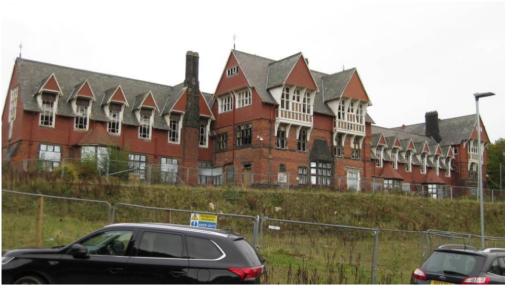
Photo 1: Cookridge Old Hospital is being converted to residential use.
